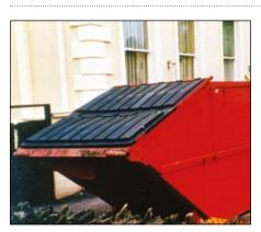
Use a lockable skip for asbestos cement sheet
